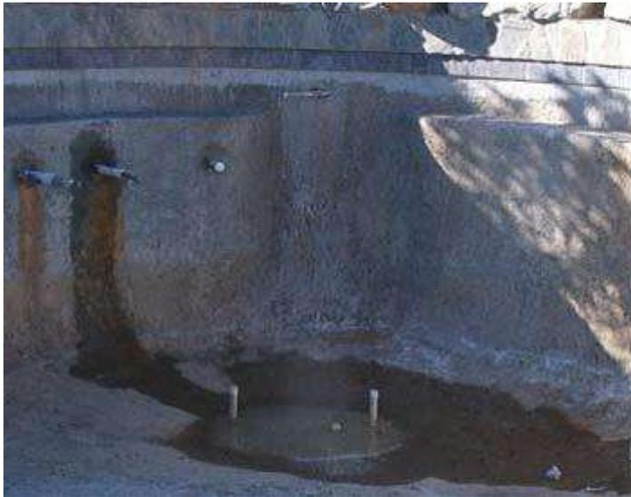
**Water intrusion at penetrations from behind the structure prior to application of the interior finish coating**
