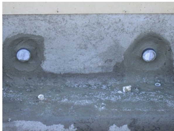
Plumbing with fittings installed and pre-sealed.
